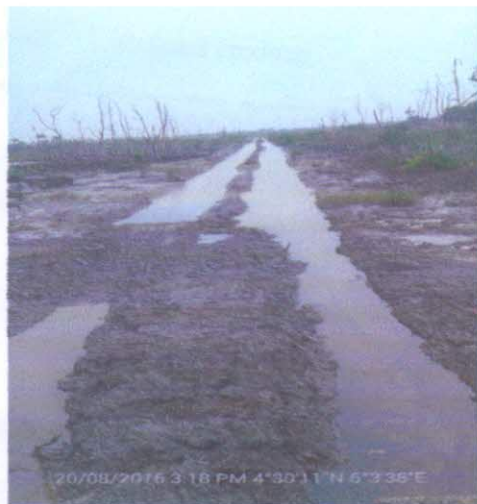
Fig D: picture taken after backfilled.
